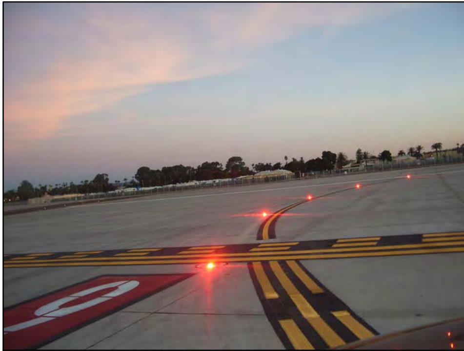
FIG 2-1-12 Runway Entrance Lights
